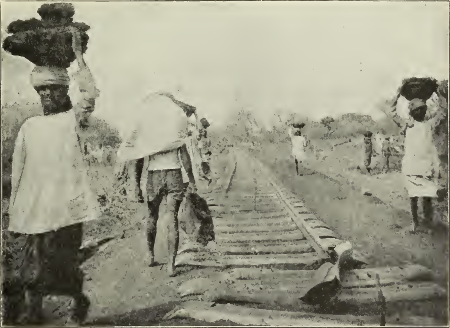
“ANOTHER GANG DROPS THE RAILS IN THEIR PLACES.”
